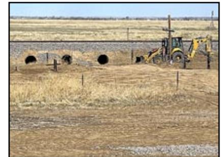
BNSF expedited replacement of the wildfire damaged trestle 5-miles west of La Junta, Colorado, on it’s Raton Subdivision at milepost 560.4. Amtrak’s Southwest Chiefs, train 3 & 4, use this route. BNSF installed culverts to replace the wildfire damaged 65-foot trestle. Culverts were in place by April 25, 2022 and Amtrak’s Southwest Chief service was reinstated. – Two Photos © 2022 by Chip.
