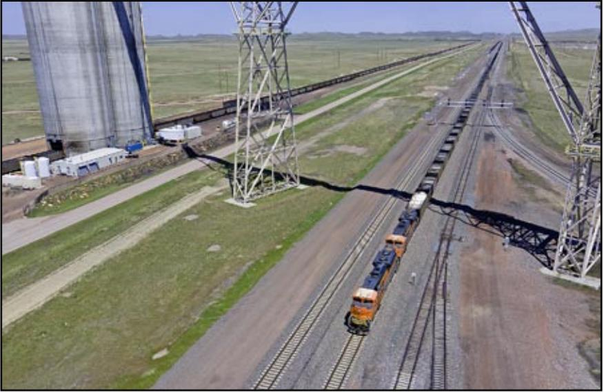
The West Black Thunder loadout was built a little over ten years ago, and the sheer scale of the loadout is impressive. A conveyor belt system brings coal from the actual mine, several miles to the east. The conveyor belt rises up and over the triple track main and into the massive concrete tipple. In this shot, a train loads underneath said tipple, while two SD70ACes bring up the tail end of a westbound empty on Main 2. – Photo © Kevin Morgan.
