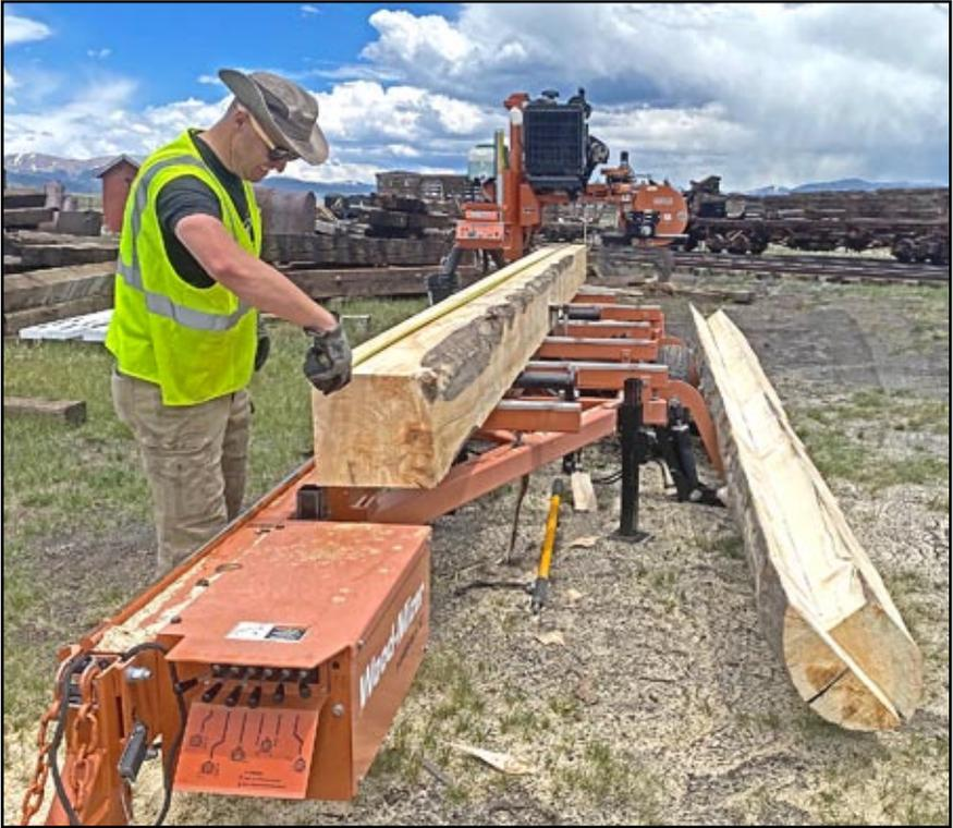
One of the main timbers for the new Como tank base being milled to size at Como. – Photo courtesy South Park Rail Society and the DSP&PHS.
