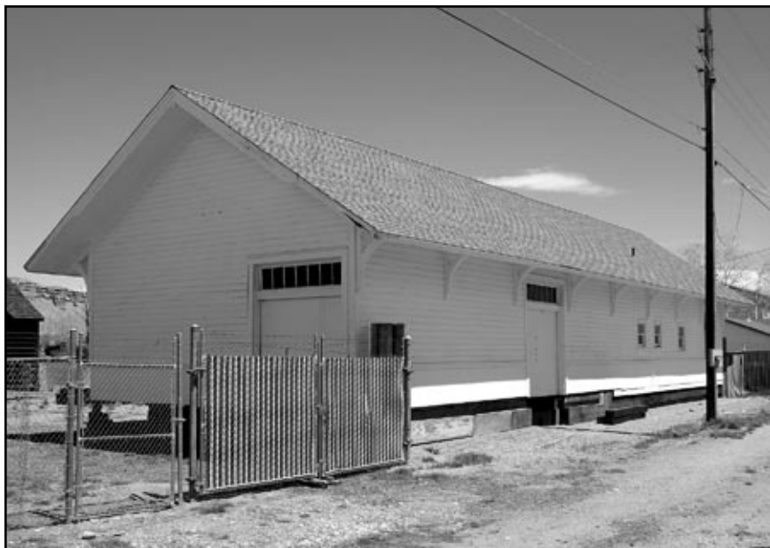
The historic 1906 Moffat Road (DNW&P) depot at the Heritage Park Museum in Kremmling, Colorado, with the new permanent, fake shingle roof thanks to the grant from the UP Foundation. – Photo © 2009 Jim Yust.
