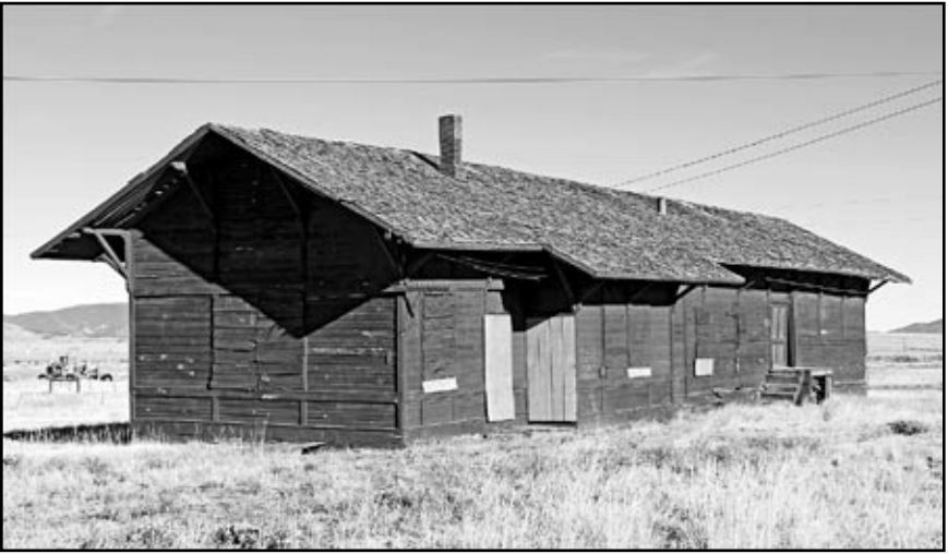
The Colorado Midland depot still stands at Hartsel, Colorado, on November 29, 2011. – Photo © 2011 Dave Schaaf.
