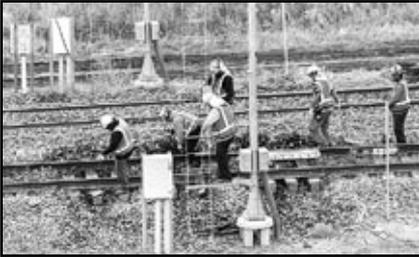
The tie plate gang follows behind and positions the tie plates for the tie plate inserter, kicks away ballast and uses sledge hammers to fine-tune the positioning of the ties. A tamper machine lifts ties to bottom of the rails.
