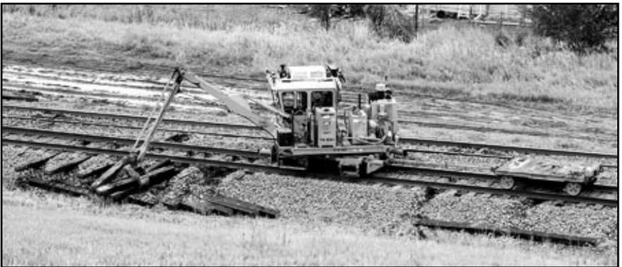
The resulting hole for the new ties is deepened by an augur, and two machines that follow partially insert the new tie about half way in – their hydraulics are not strong enough to push the new tie fully into place. – Photo © 2017 Linda Fike.
