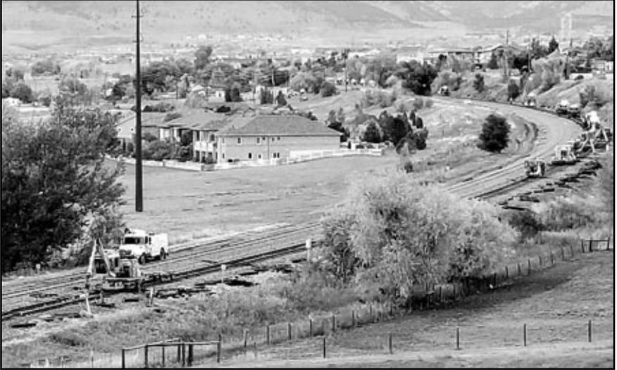
The following is a team effort description of the process as it unfolded: Initially, two machines remove spikes, with workers following to pull tie plates and knock out rail anchors. They are followed by two machines that remove the ties and lay them along the right of way. – Photo © 2017 Linda Fike.
