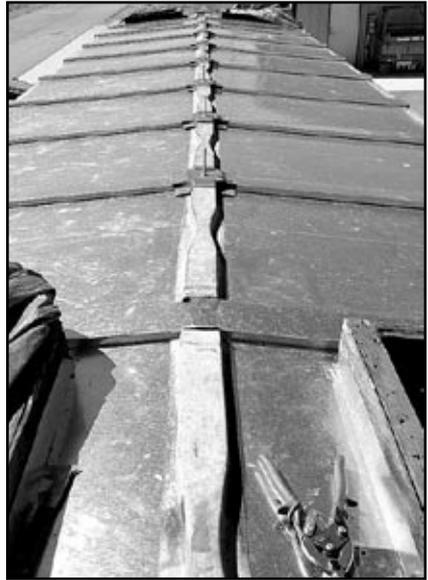
New galvanized roof panels and seam covers fabricated and installed by Holt Sheet Metal. The old ridge pieces were reused.
